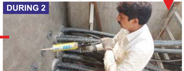
3) Cable Sealing With Fst250 Application
