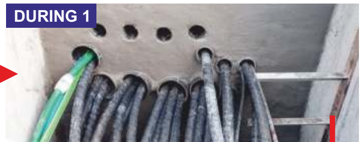
3) Cable Sealing With Fst250 Application
